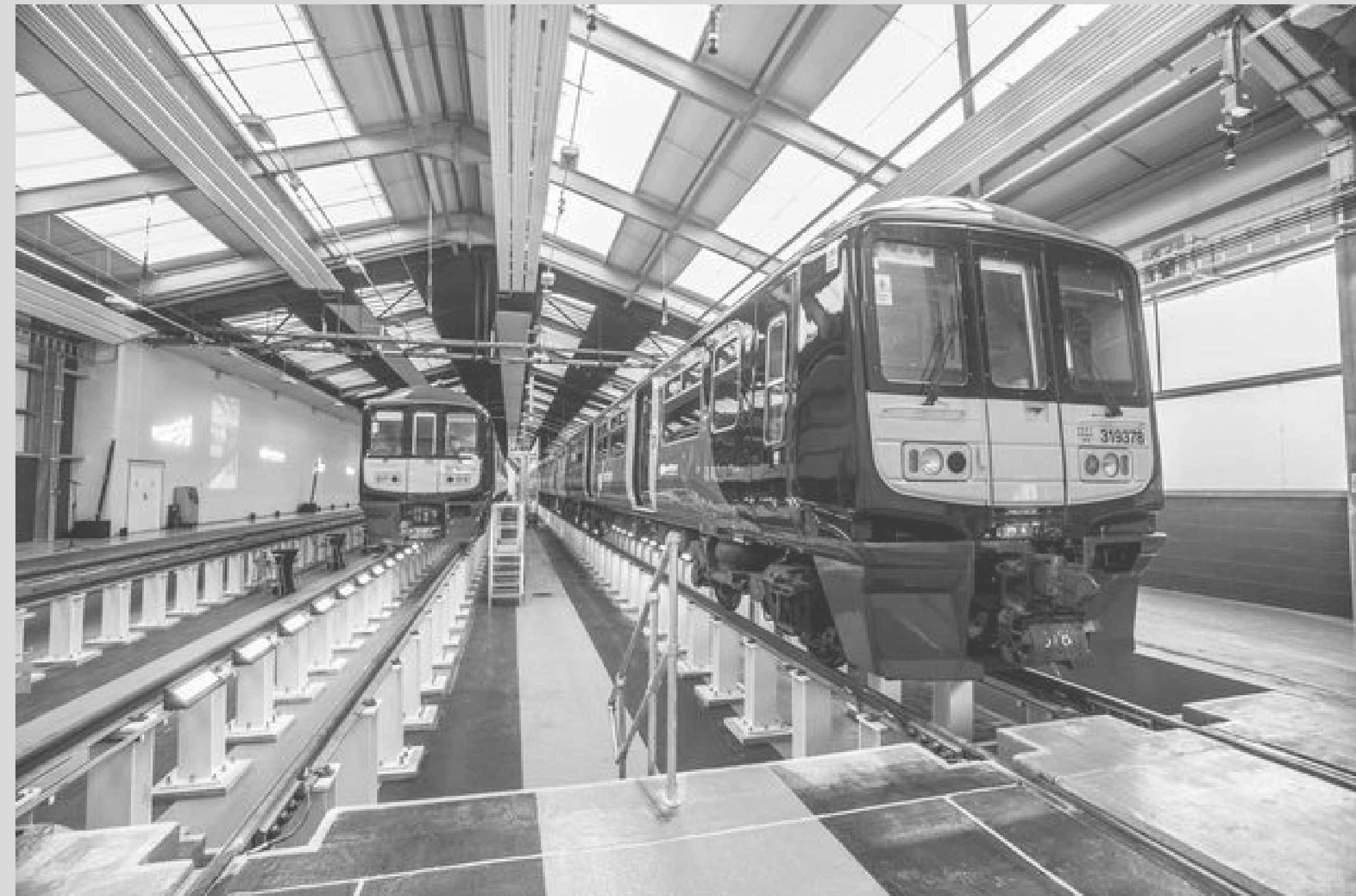
Special track forms in Depot Areas
